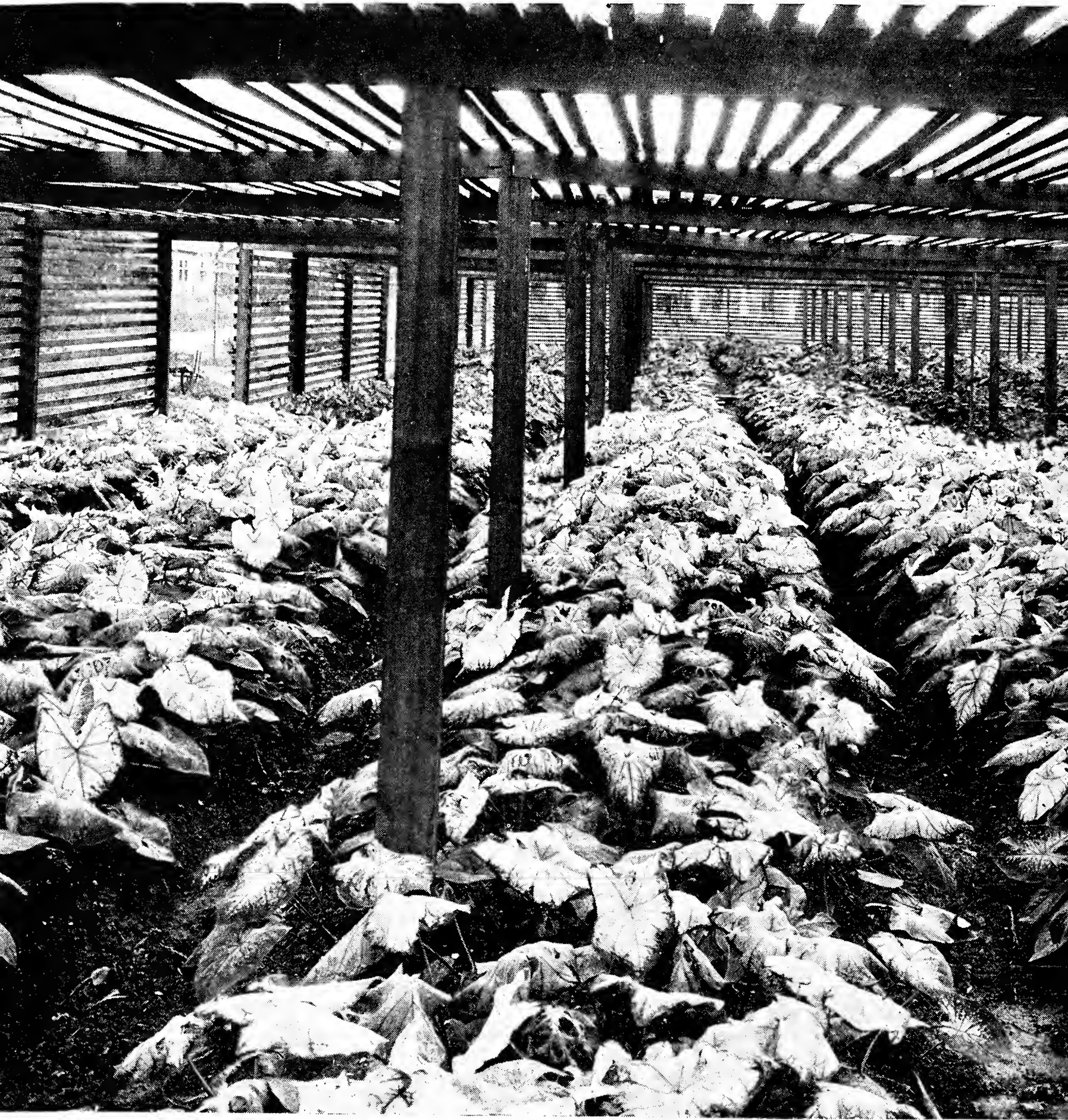
Section One of Reuter's Caladium Lathhouse
